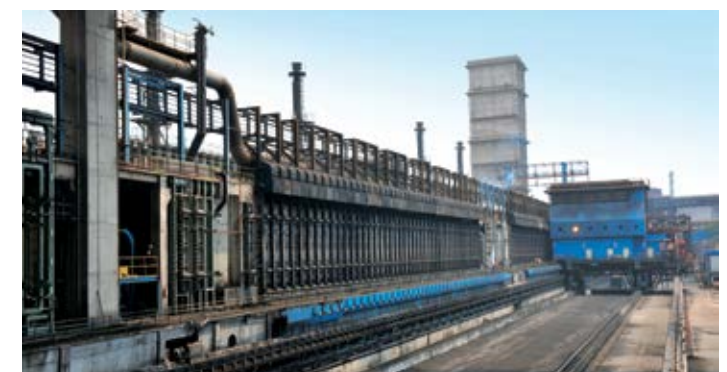
Coke oven battery executed by L&T for one of India's major steel plants.
