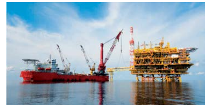
L&T's heavy-lift-cum-pipelay vessel LTS 3000 installing a topside for Newfield Peninsula in Malaysia.
