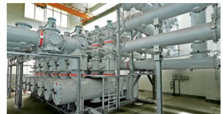
One of many 400 kV gas-insulated substations (GIS) installed by L&T. Currently it is executing India's first 765 kV GIS in Pune.
