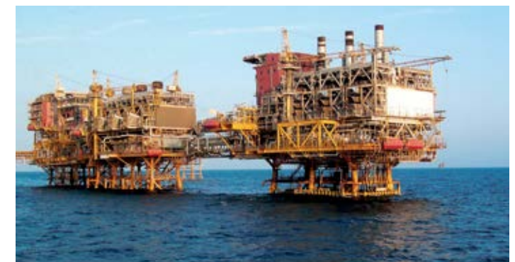
Booster compressor platform with an interconnecting bridge, built by L&T for Oil & Natural Gas Corporation (ONGC) in South Basin Gas Fields.
