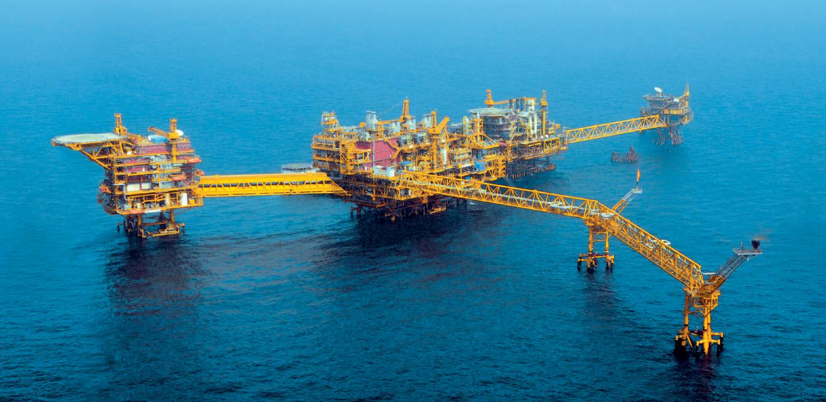
Mumbai High North Complex of ONGC, executed by L&T on an EPC basis. The massive complex comprises a process platform, a living quarters platform & control room, three process gas compression platforms, two flare platforms and two jackets including one weighing 13,500 tonnes.
