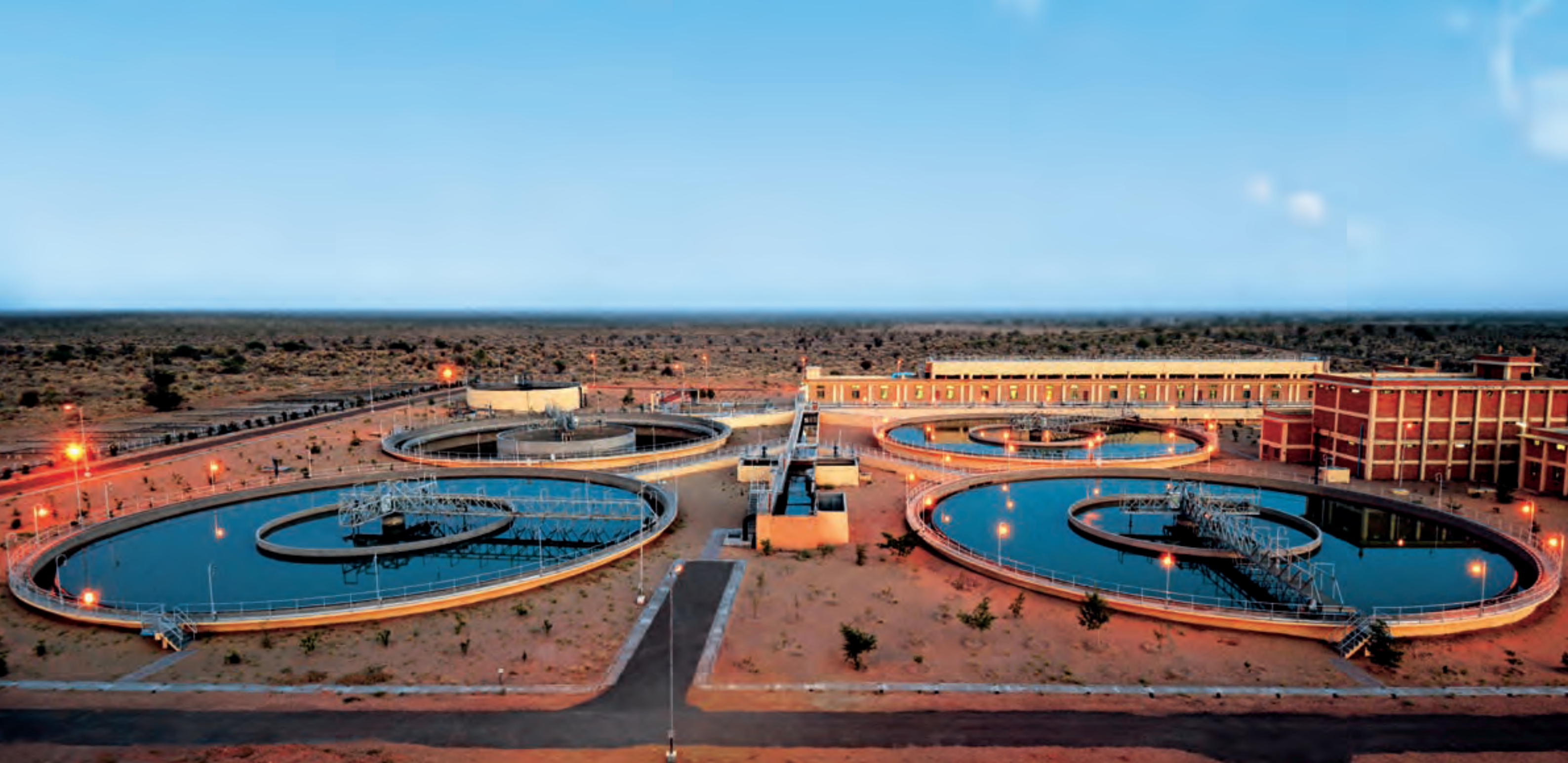
172 MLD water treatment plant for Barmer Lift Water Supply Project at Jaisalmer, Rajasthan. L&T has designed and constructed water reservoirs, pumping stations, pipeline networks and distribution systems.
