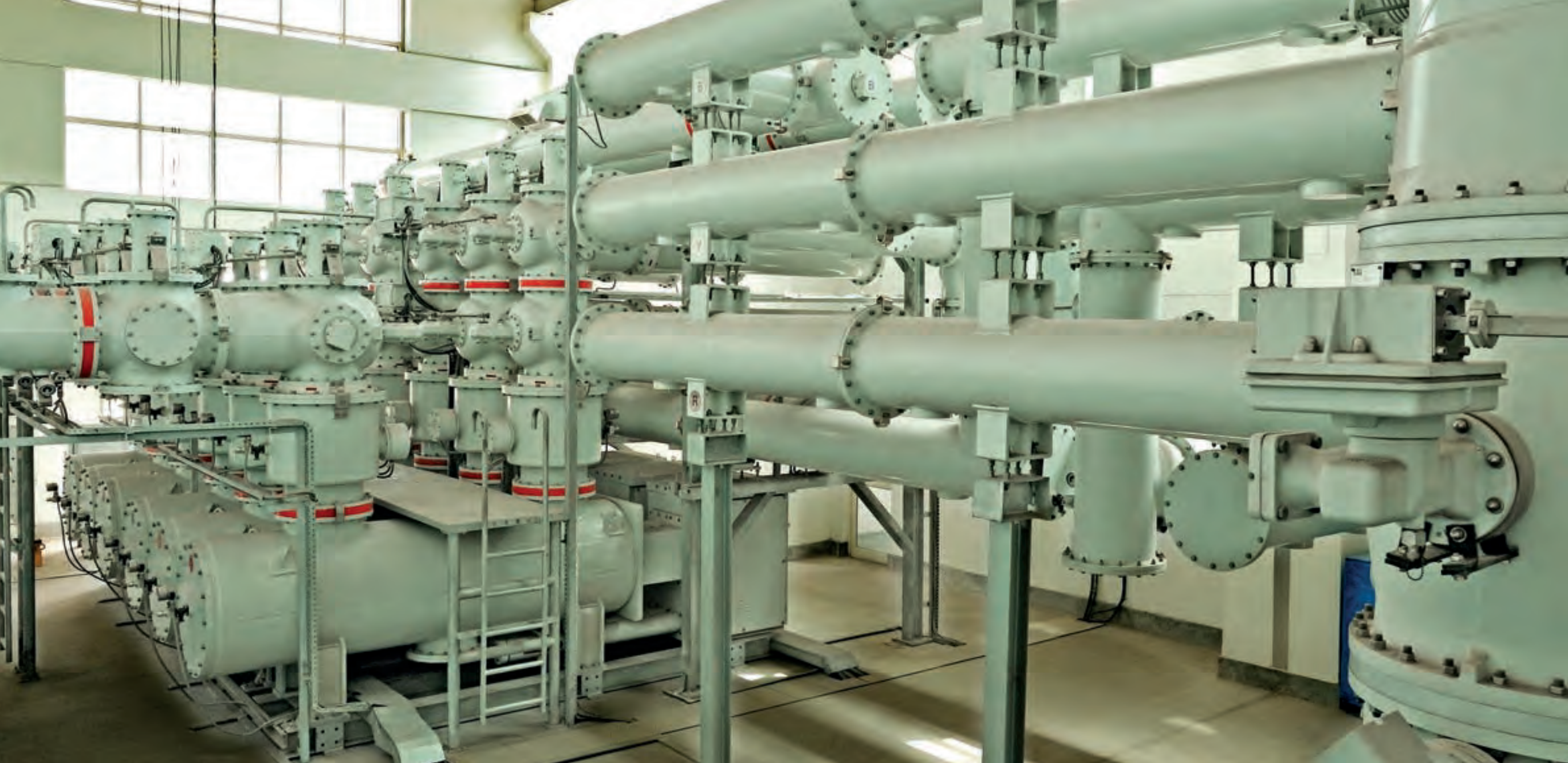
One of many 400 kV Gas-Insulated Substations (GIS) installed by L&T. The Company is one of the major players in the power transmission and distribution sector in the Middle East, with a track record extending across the UAE, Qatar, Kuwait, Oman and Saudi Arabia.
