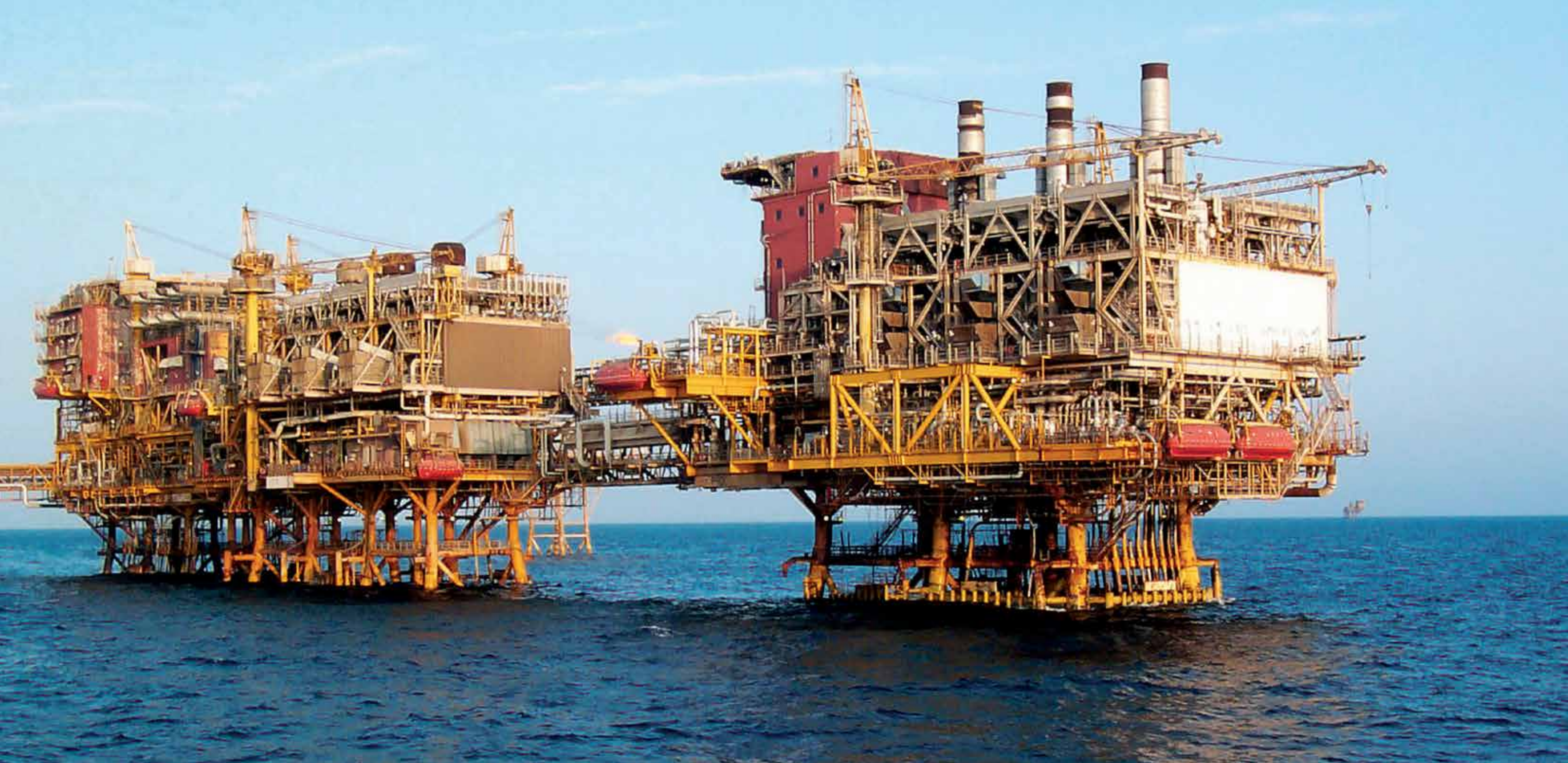
Booster compressor platform with an interconnecting bridge executed for Oil & Natural Gas Corporation (ONGC) in South Basin Gas Fields off India's west coast. This project won the 'PMI Distinguished Project Award' from Project Management Institute, USA.
