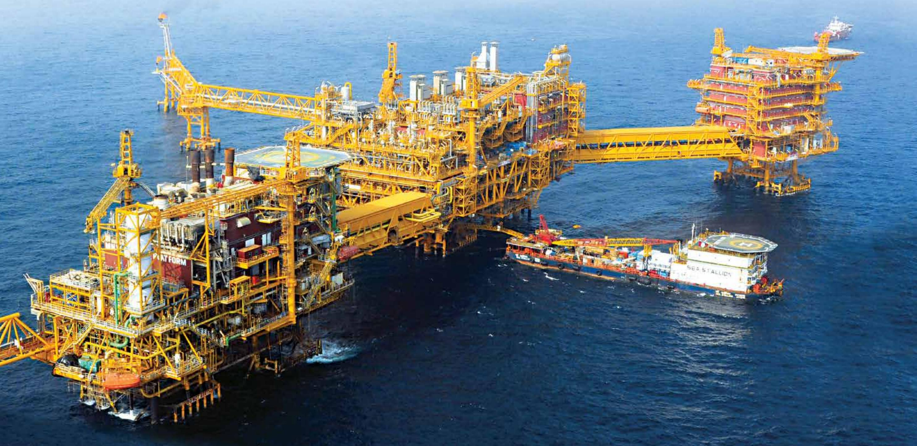
Mumbai High North (MHN) Complex of ONGC, executed on EPCI basis. The massive complex comprises a process platform (26,500 MT Topside + 13,500 MT Jacket), a living quarters platform (6,500 MT Topside + 13,500 MT Jacket), two flare platforms and four bridges.
