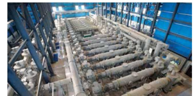
India's first 765 kV gas insulated substation at Pune.
