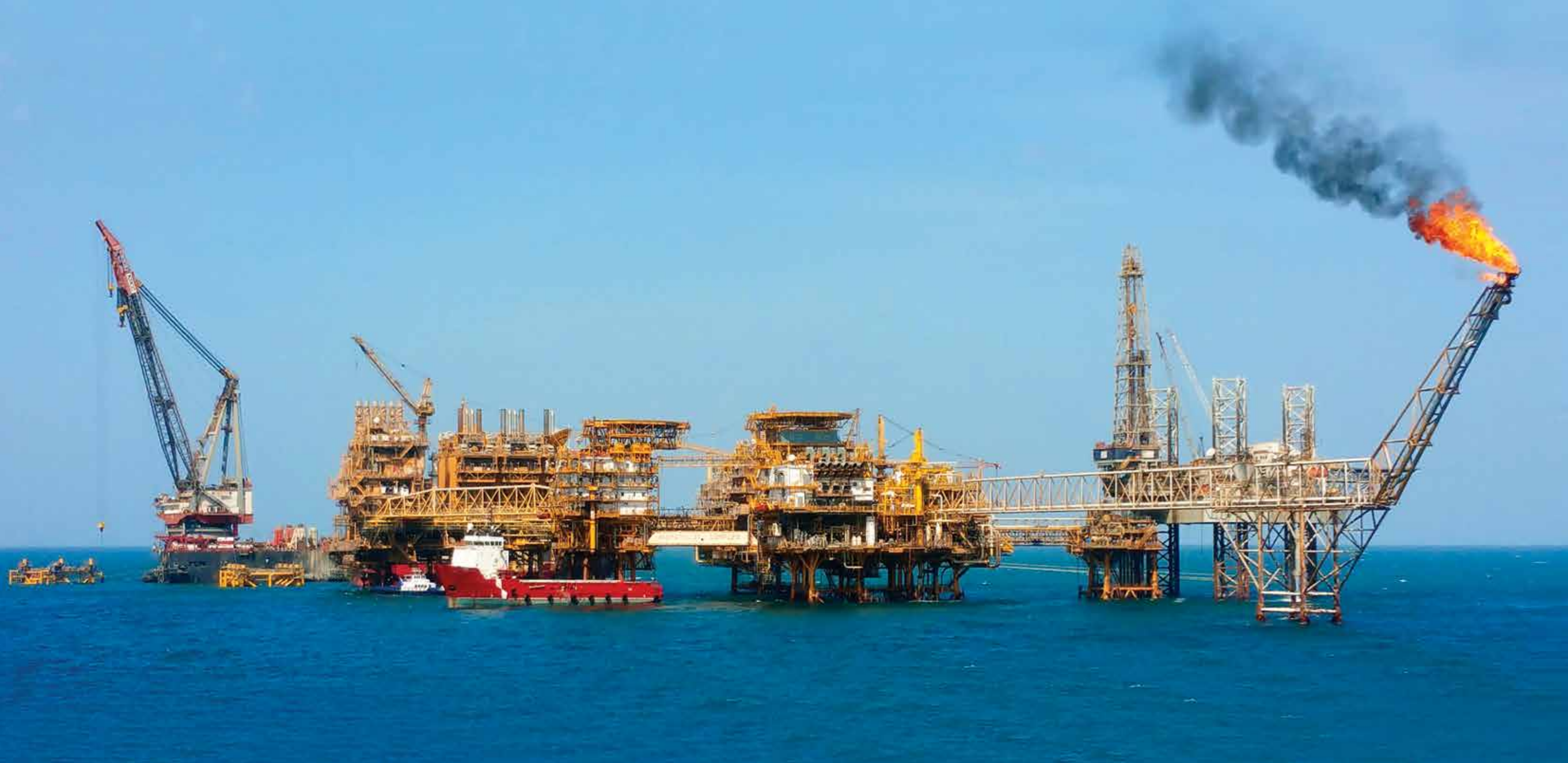
Bassein Development Project for ONGC. The scope included BCPA3 process platform, BLQ3 Living Quarters platform, BH wellhead platform, 12 km pipelines, bridges and modifications at BPA complex.
