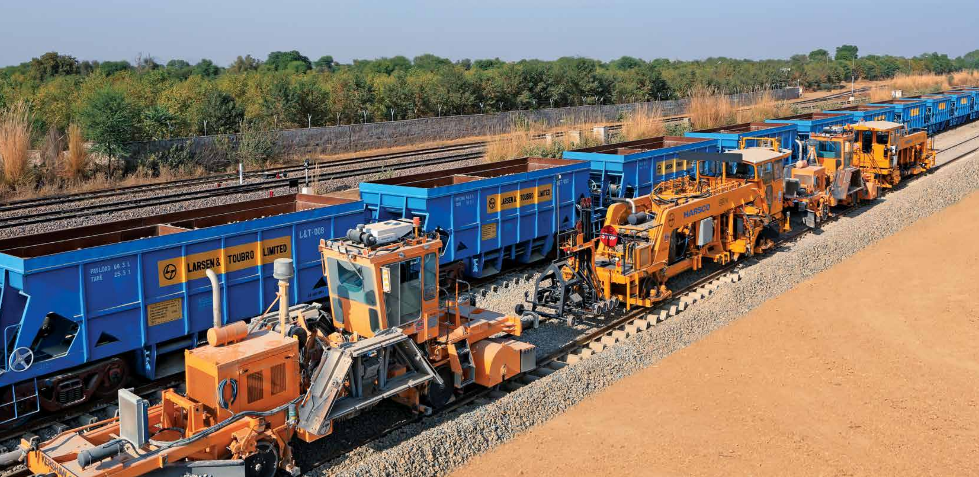
Capable of laying 2 km of tracks per day, the new track construction machine, owned by L&T, sets a benchmark in high-speed rail construction on the Western Dedicated Freight Corridor project. L&T is currently executing a number of prestigious railway projects in India and the GCC region.
