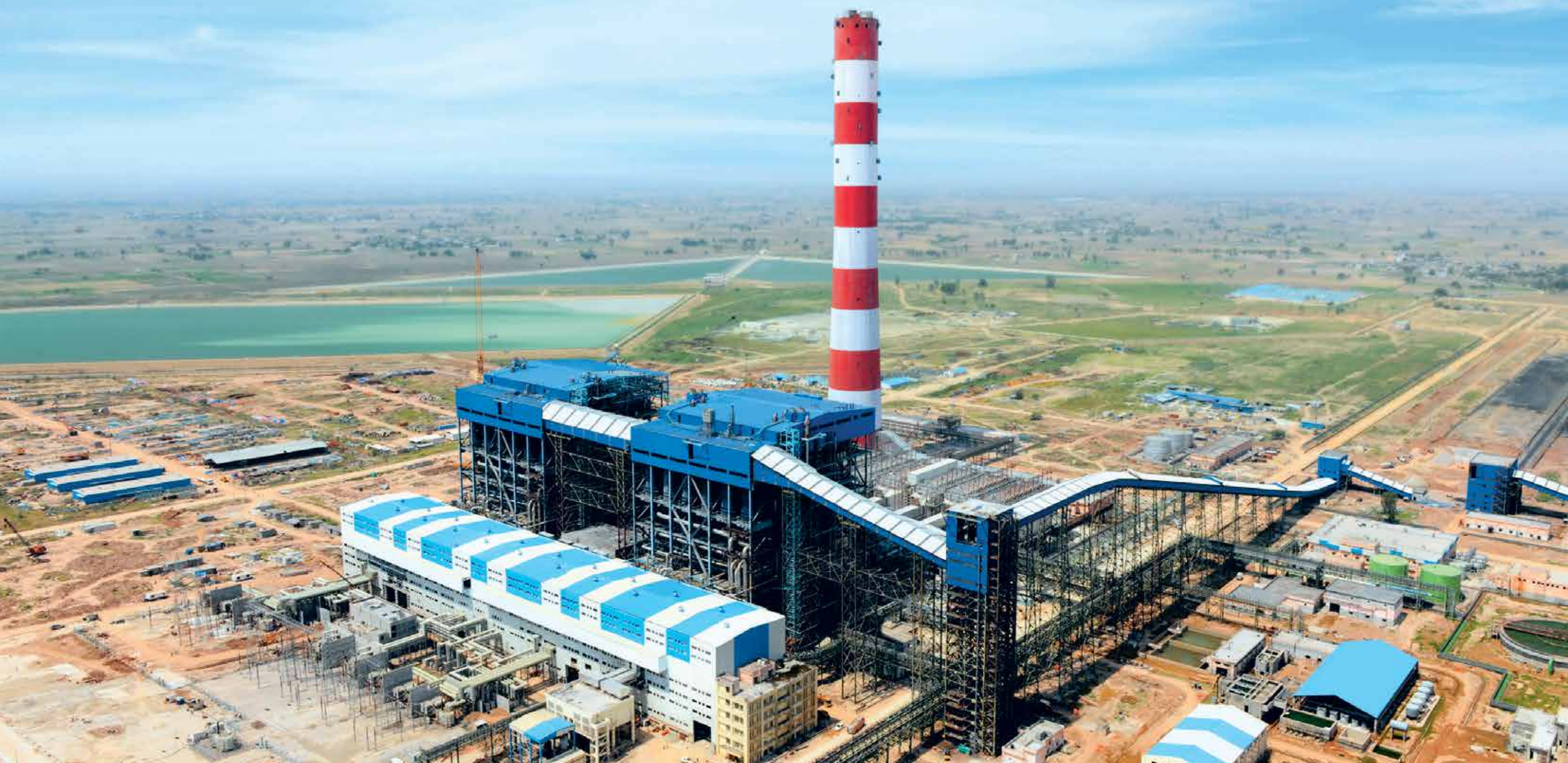
First supercritical coal-fired power project (full EPC) by L&T - 2x700 MW Supercritical Thermal Power Plant for Nabha Power Ltd at Rajpura, Punjab. L&T has manufactured critical equipment like turbine-generators, boilers, ESPs and axial fans, among other systems, for supercritical power plants across India.
