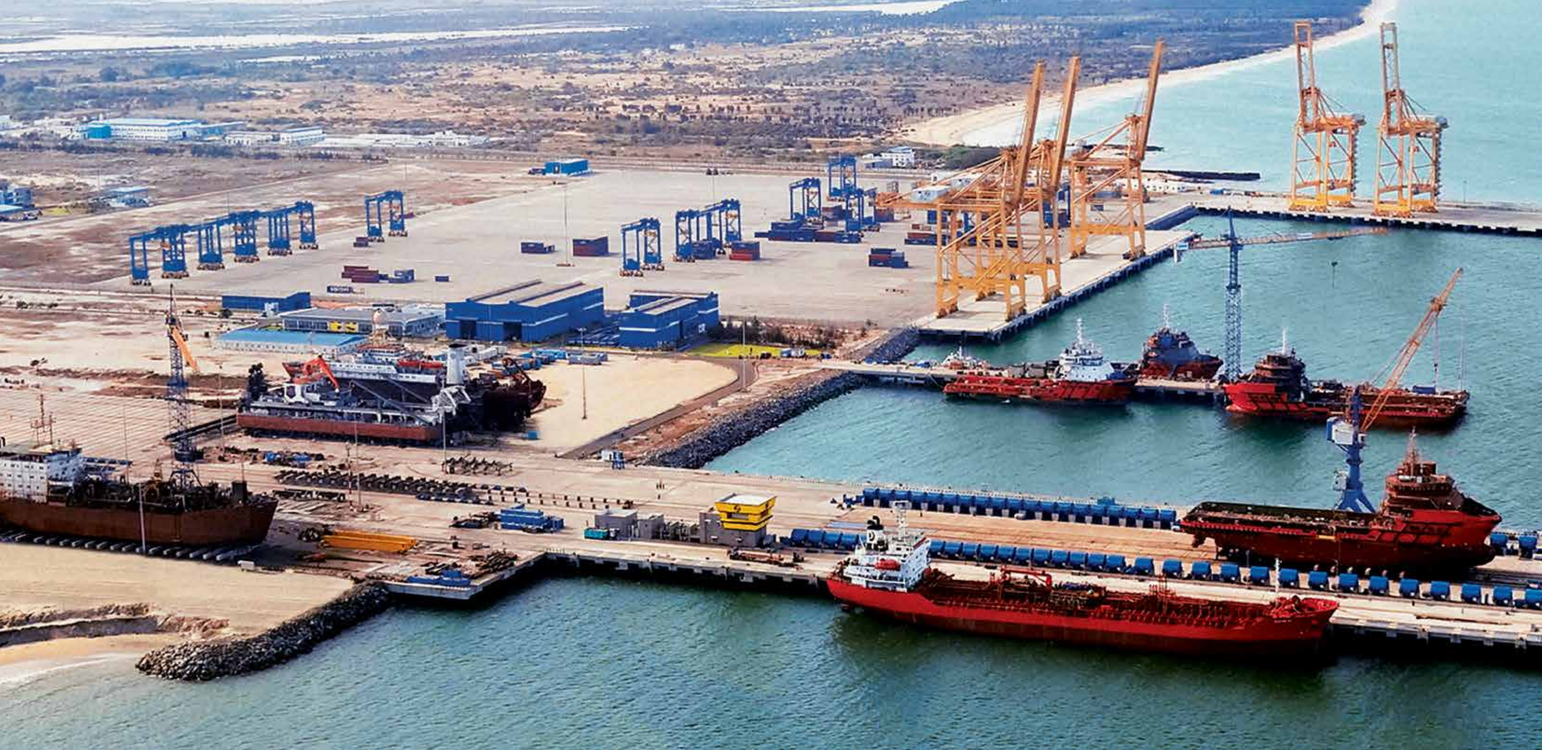
L&T's shipyard at Kattupalli on India's east coast – equipped with a shiplift, designed and built in-house. L&T undertakes ship design, building, maintenance and repair services for a wide range of defence vessels.
