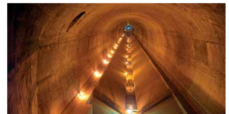
Huge desilting chambers – part of Bhutan's largest hydel project, at Punatsangchhu.
