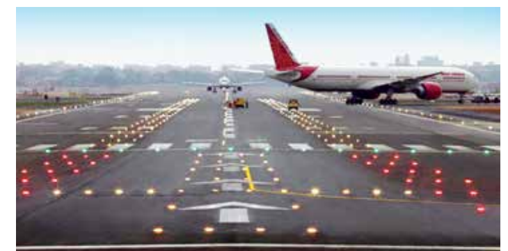
Airfield ground lighting. Runways built by L&T include those incorporating CAT III/B Instrument Landing Systems.
