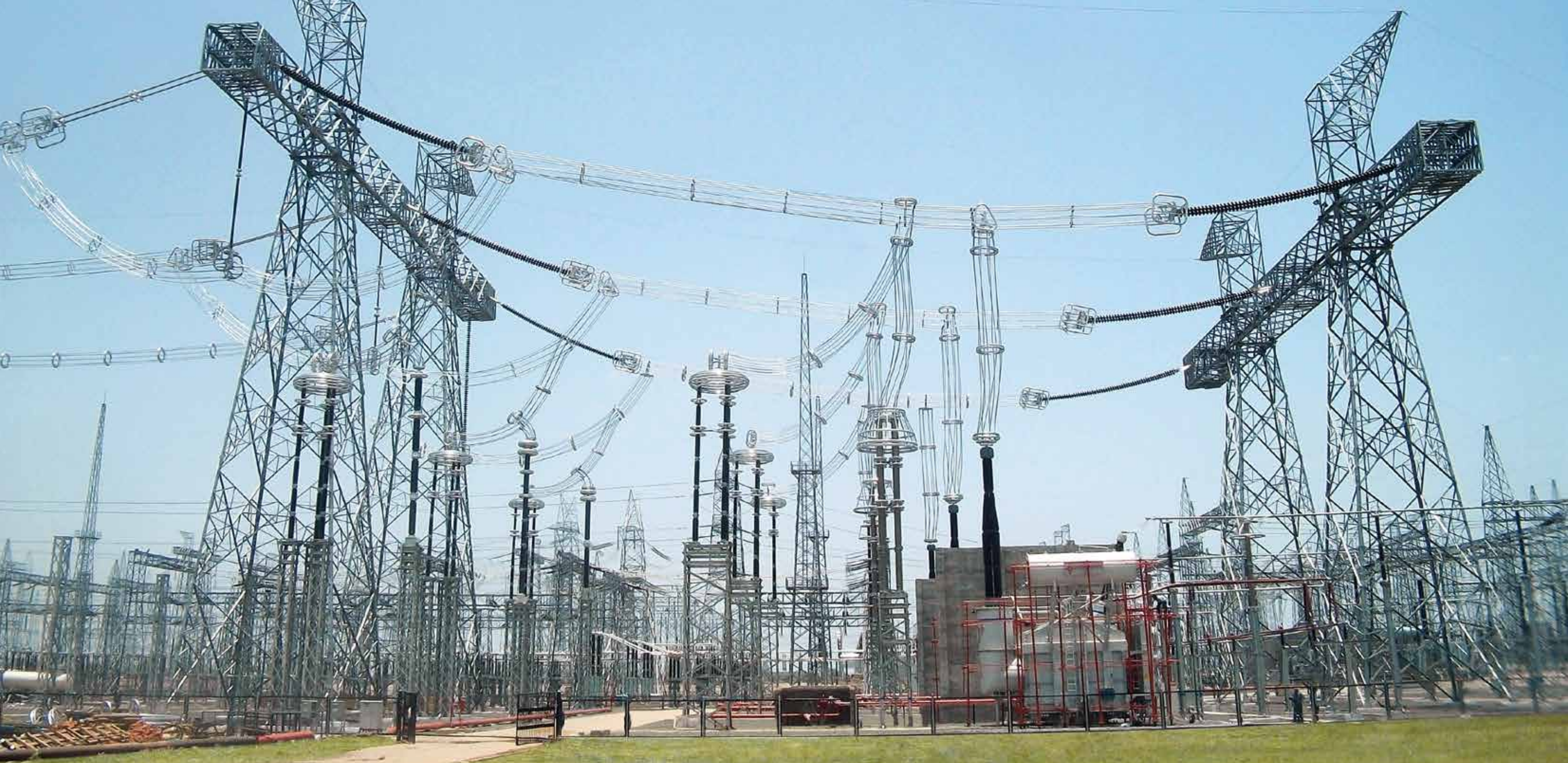
India's first 1200 kV Air-insulated Substation at Bina in Madhya Pradesh. L&T offers complete solutions in high-voltage substations and power transmission lines.
