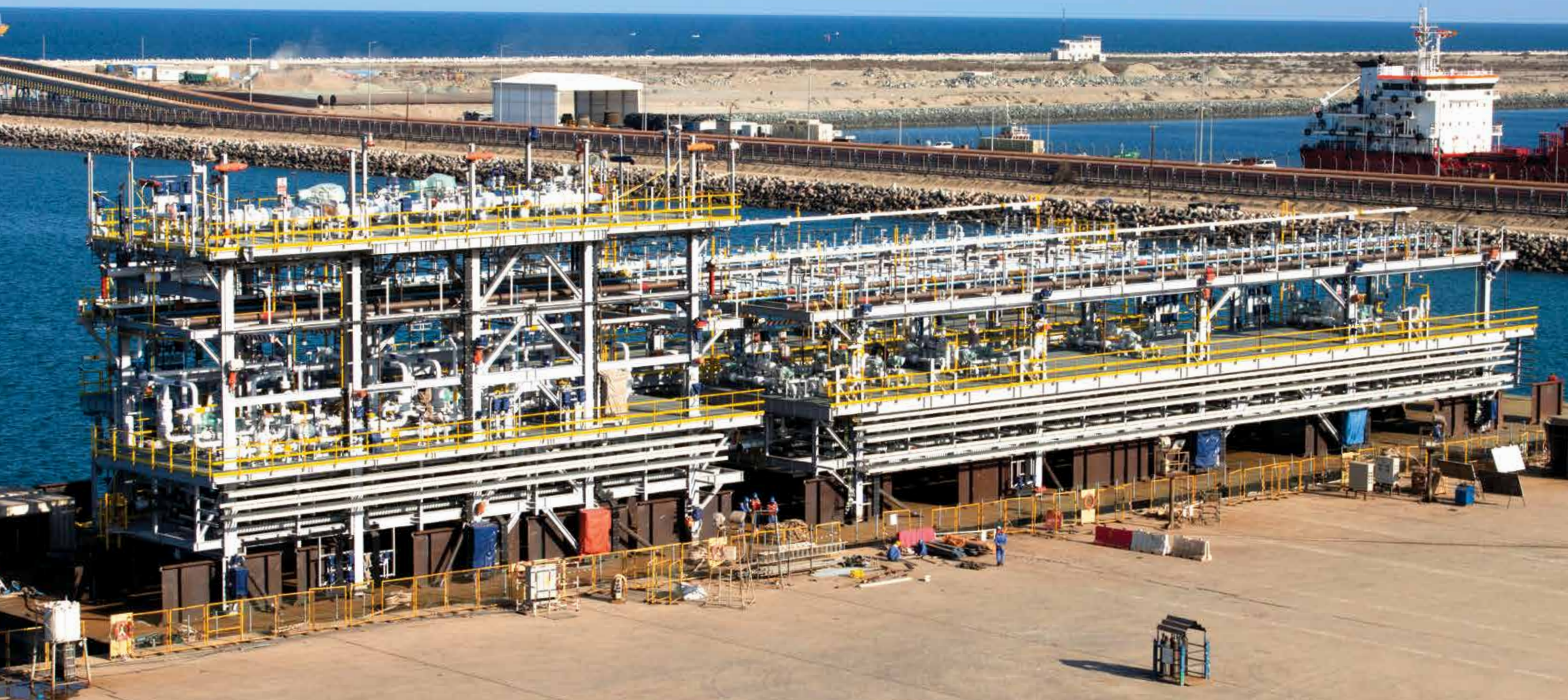
PAM and PAR modules for ExxonMobil / ZADCO's Upper Zakum Field development programme, ready for despatch at Sohar Yard in Oman. The scope includes engineering, fabrication and load-out of 33 modules weighing approx. 14,000 MT.
