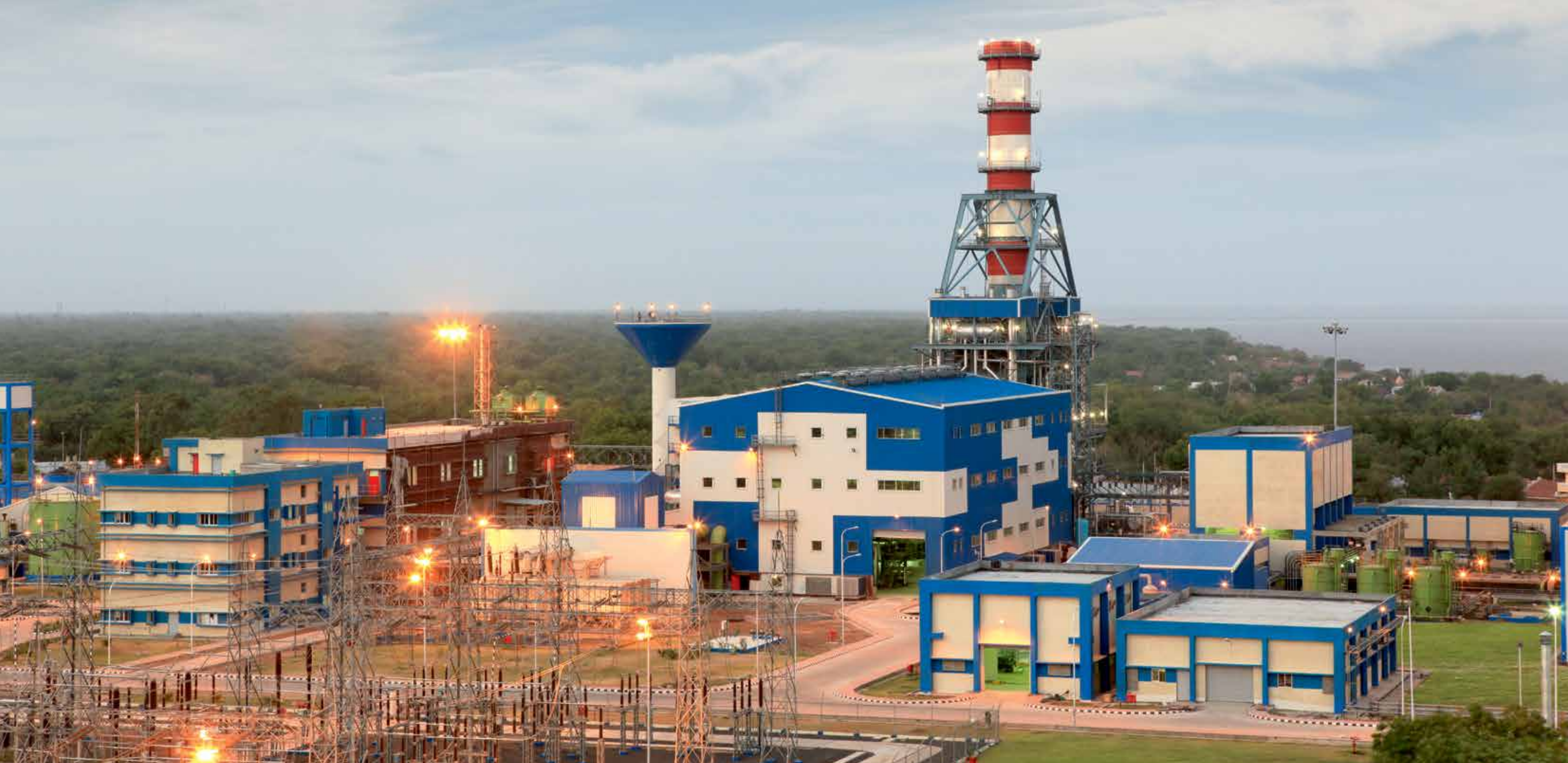
On EPC basis, L&T undertook the 375 MW single-shaft combined cycle power plant project for Gujarat State Electricity Corporation Limited at Dhuvaran.
