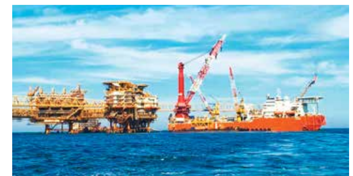
EPCIC for Additional Development of Vasai East Project for ONGC comprising 2 wellhead platforms, 35 km pipelines and modification, aided by a captive heavy lift-cum-pipelay vessel.
