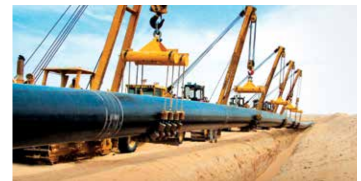
52"x 107 km Habshan-Ruwais-Shuweihat Gas Pipeline Project for GASCO, Abu Dhabi (UAE).
