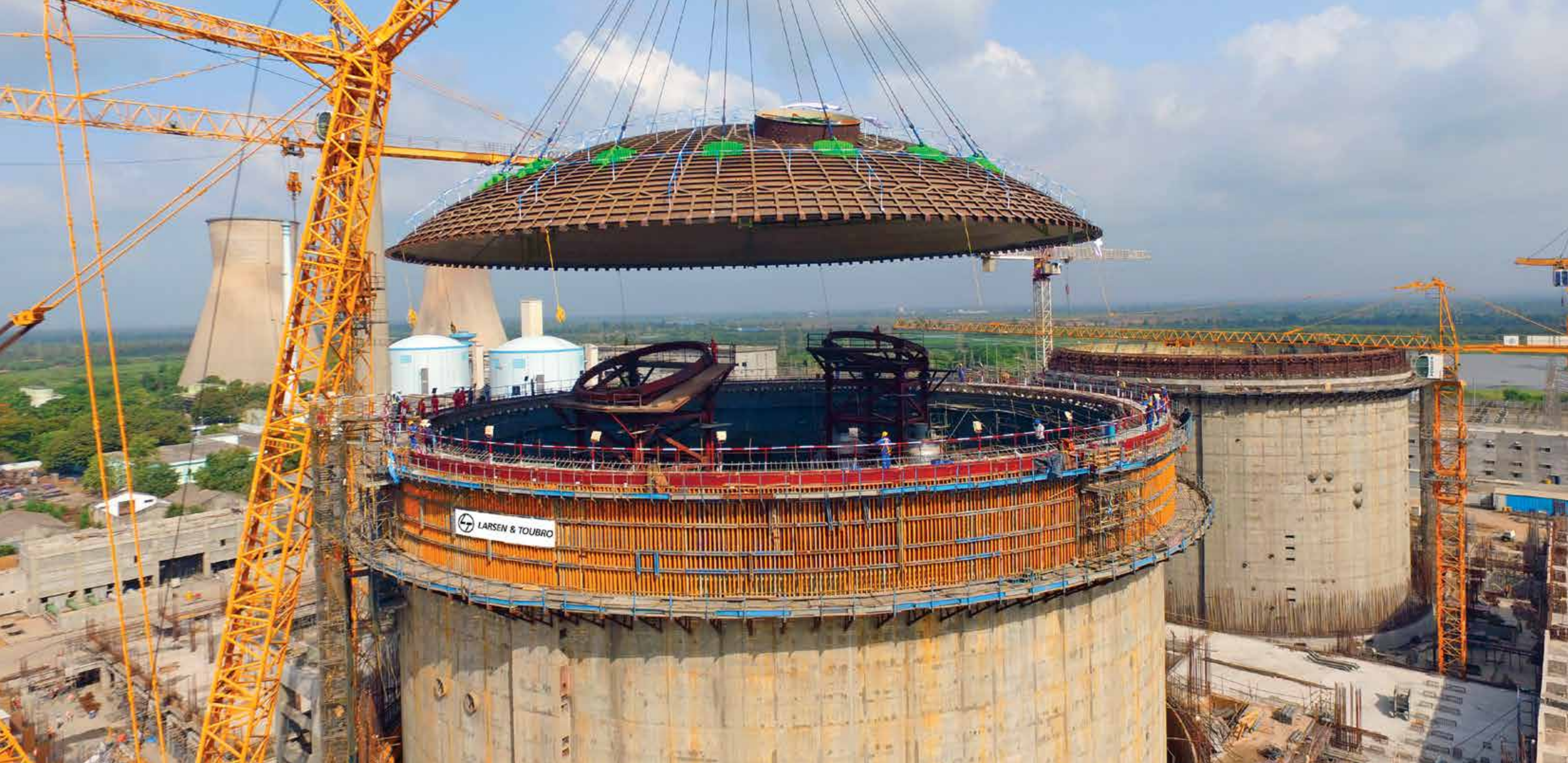
Dome erection at the Kakrapar Atomic Power project, Gujarat – the latest in L&T's five-decade association with the Nuclear Power Corporation of India. L&T has been associated with almost all of India's nuclear plants, and has expertise in both technologies – pressurised heavy water and light water.
