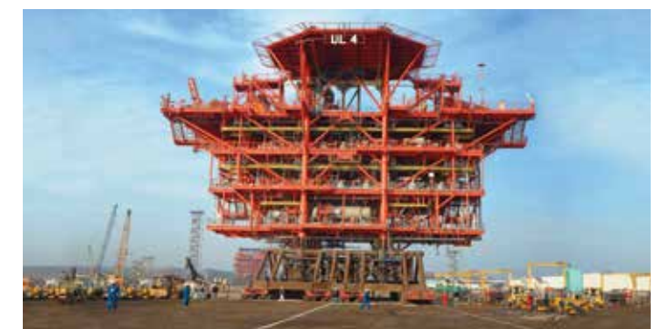
Load-out of offshore modules for ADMA-OPCO, Abu Dhabi from Sohar Yard in Oman – one of L&T Hydrocarbon Engineering's three Modular Fabrication Facilities.
