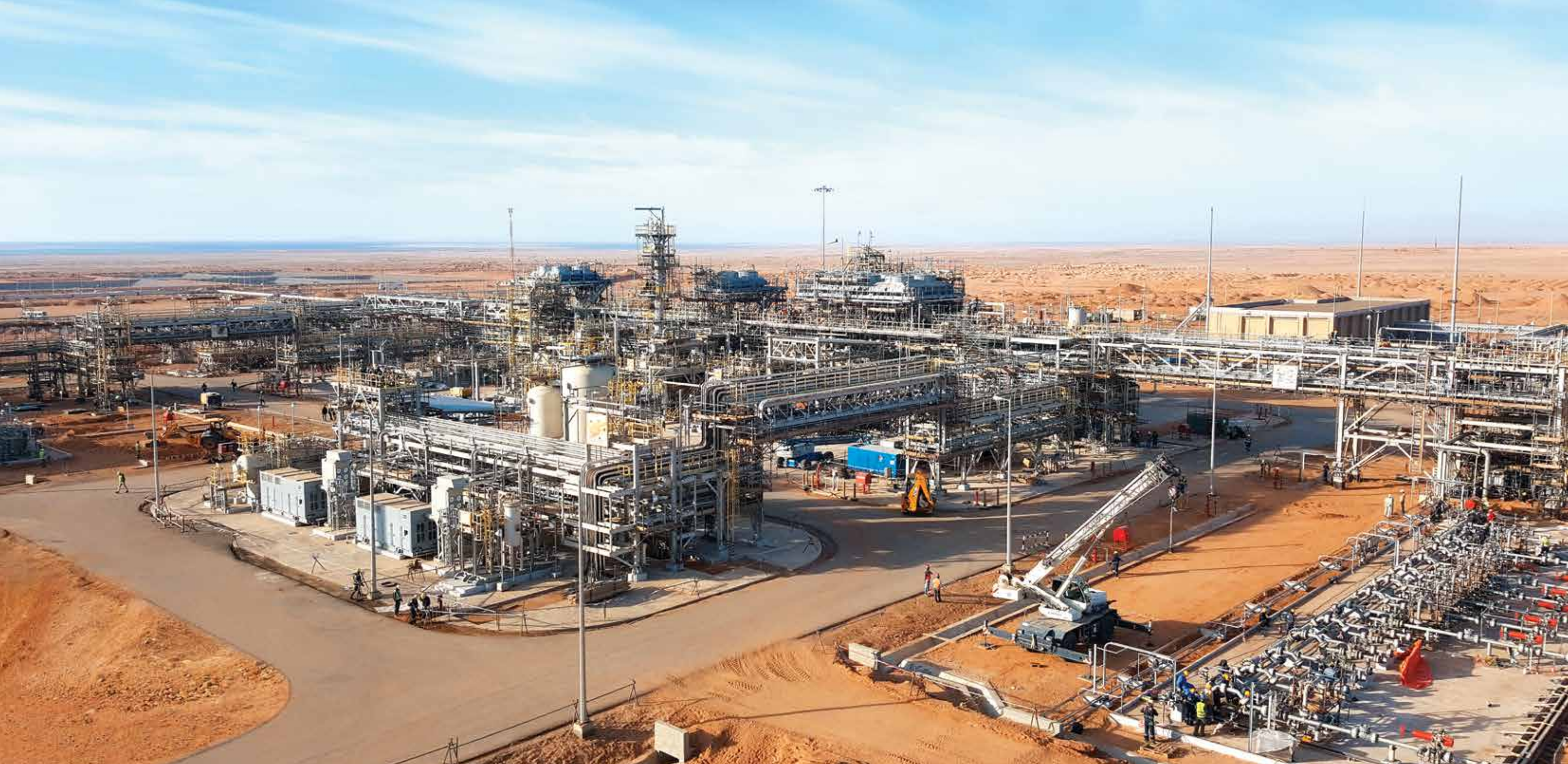
Gas processing facilities for Saudi Aramco near Tabuk in Saudi Arabia, with a capacity to treat 75 MMSCFD of gas and 4500 BPD of condensate, and the laying of over 90 km of gas and condensate product pipelines.
