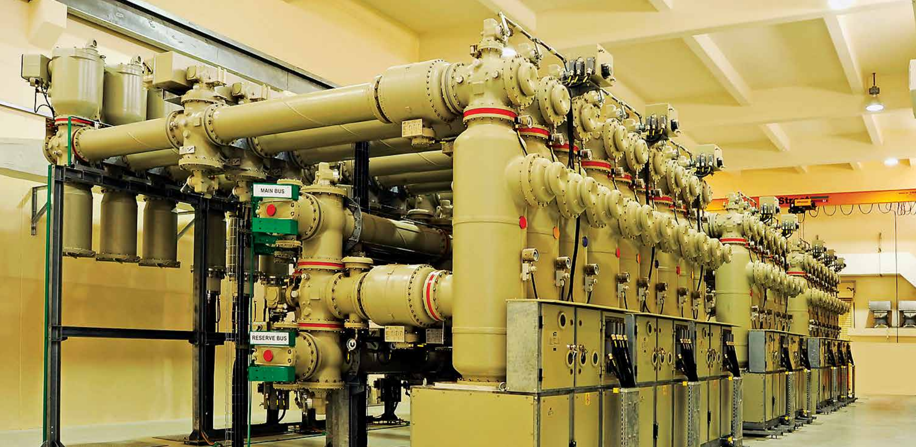
One of the many 400 kV Gas-insulated Substations installed by L&T. The Company has a track record in the power transmission and distribution sector extending across UAE, Qatar, Kuwait, Saudi Arabia, the ASEAN region and Africa.
