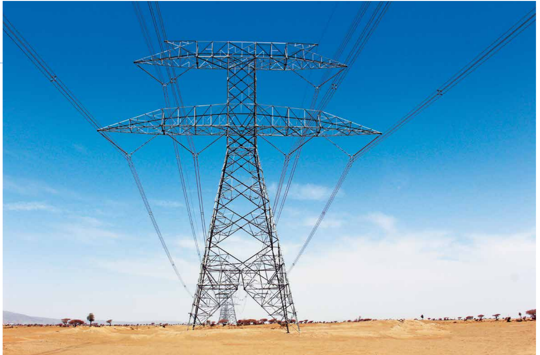
400 kV Ibri-Izki Transmission Line, Oman
