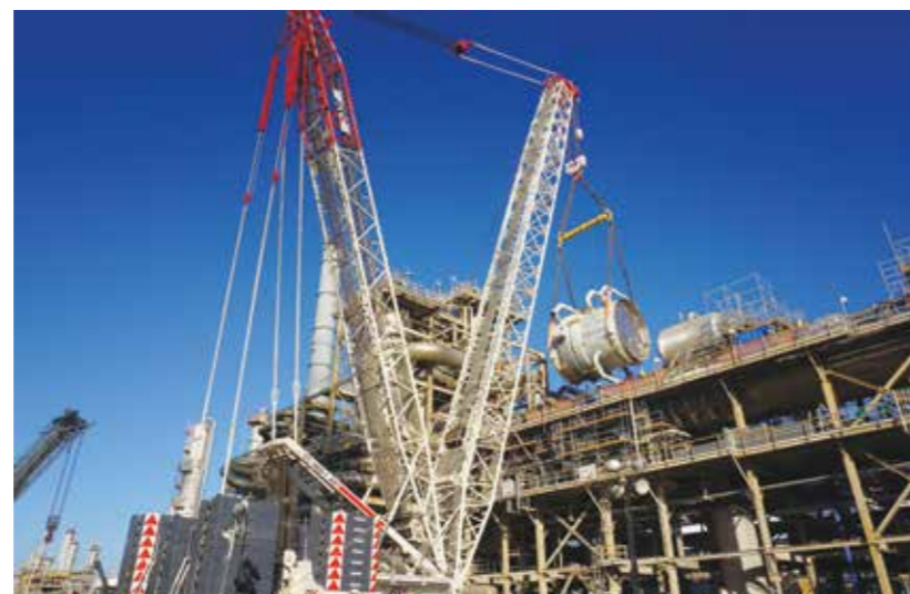
MRU - Critical Heat Exchanger Replacement at Kuwait
