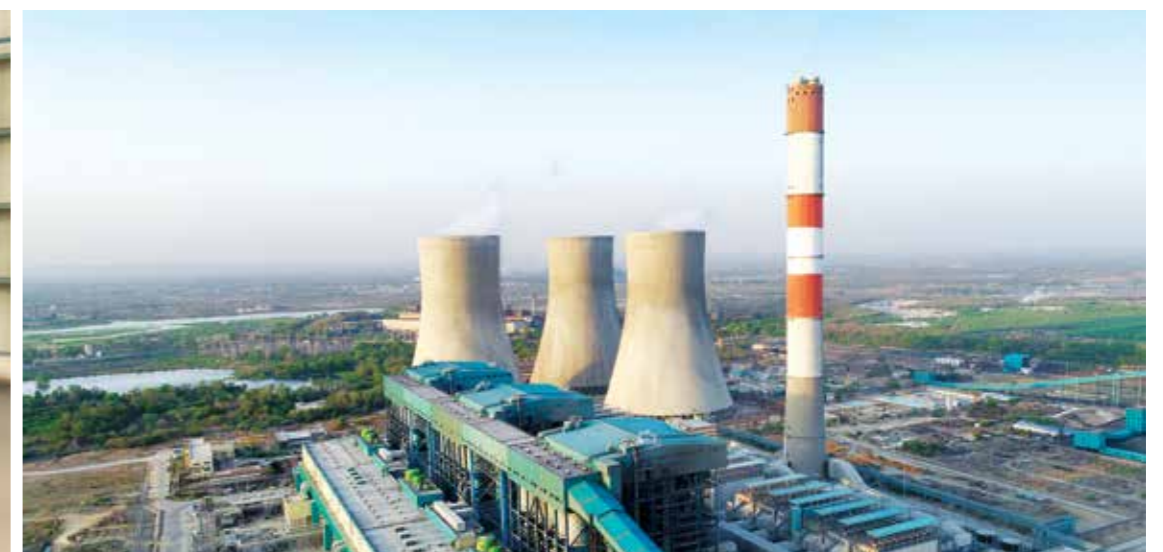
3x660 MW Koradi Thermal Power Plant, Maharashtra
