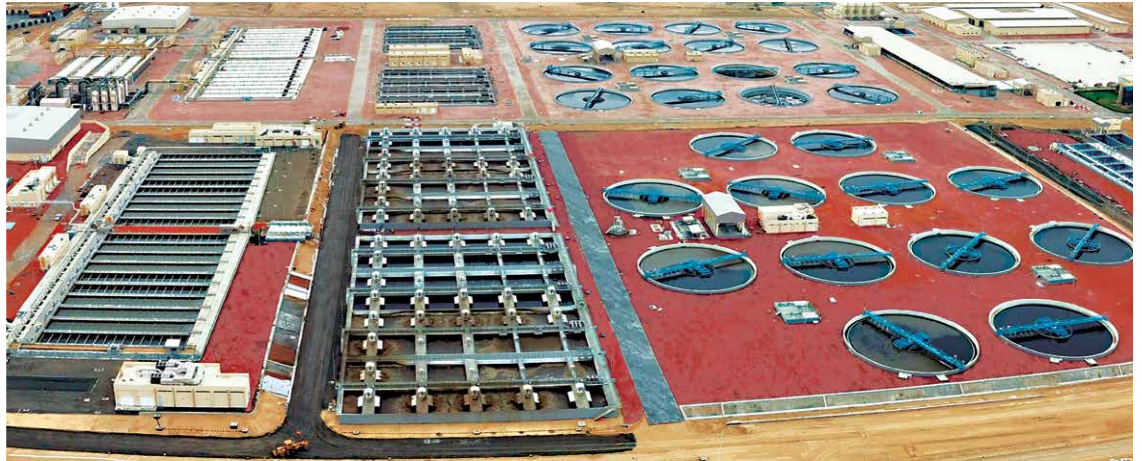
375 MLD Sewage Treatment Plant, Jebel Ali, UAE
