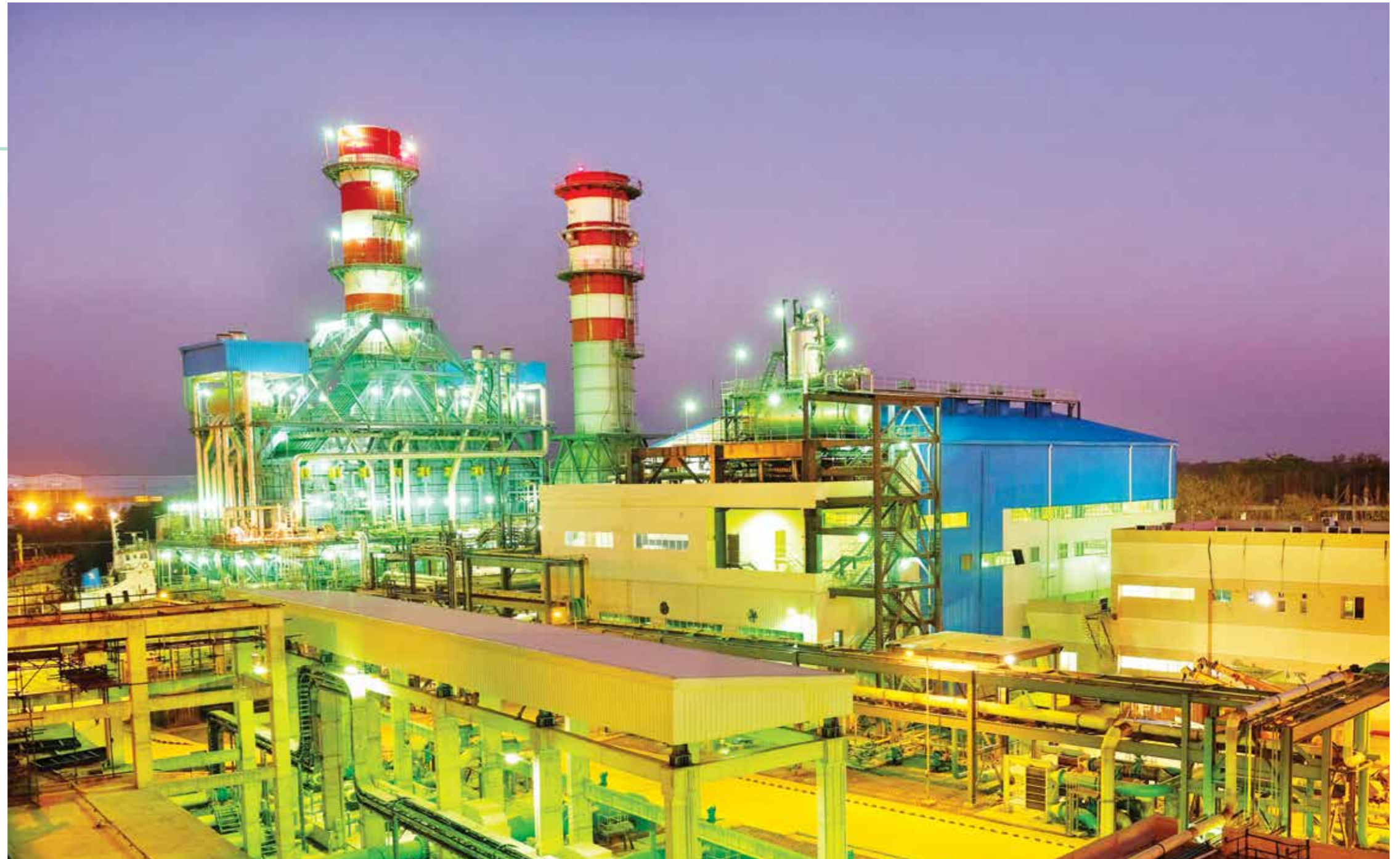
225 MW Sikalbaha Combined Cycle Power Plant, Bangladesh
