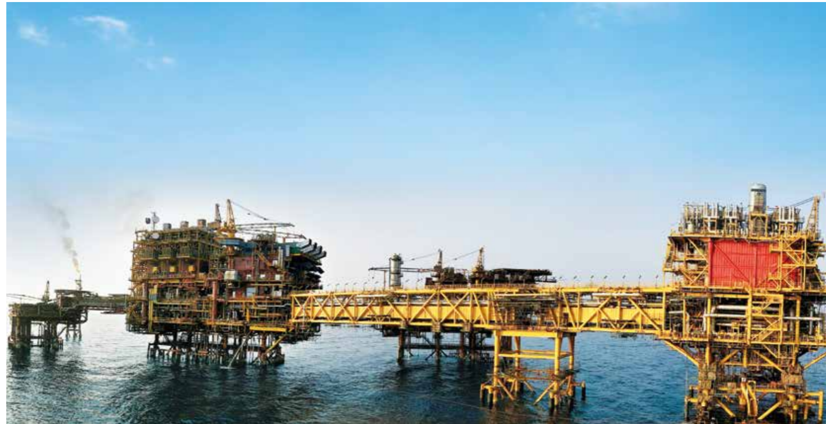
Neelam Re-development & B-173 AC Project executed for ONGC, on EPCIC basis
