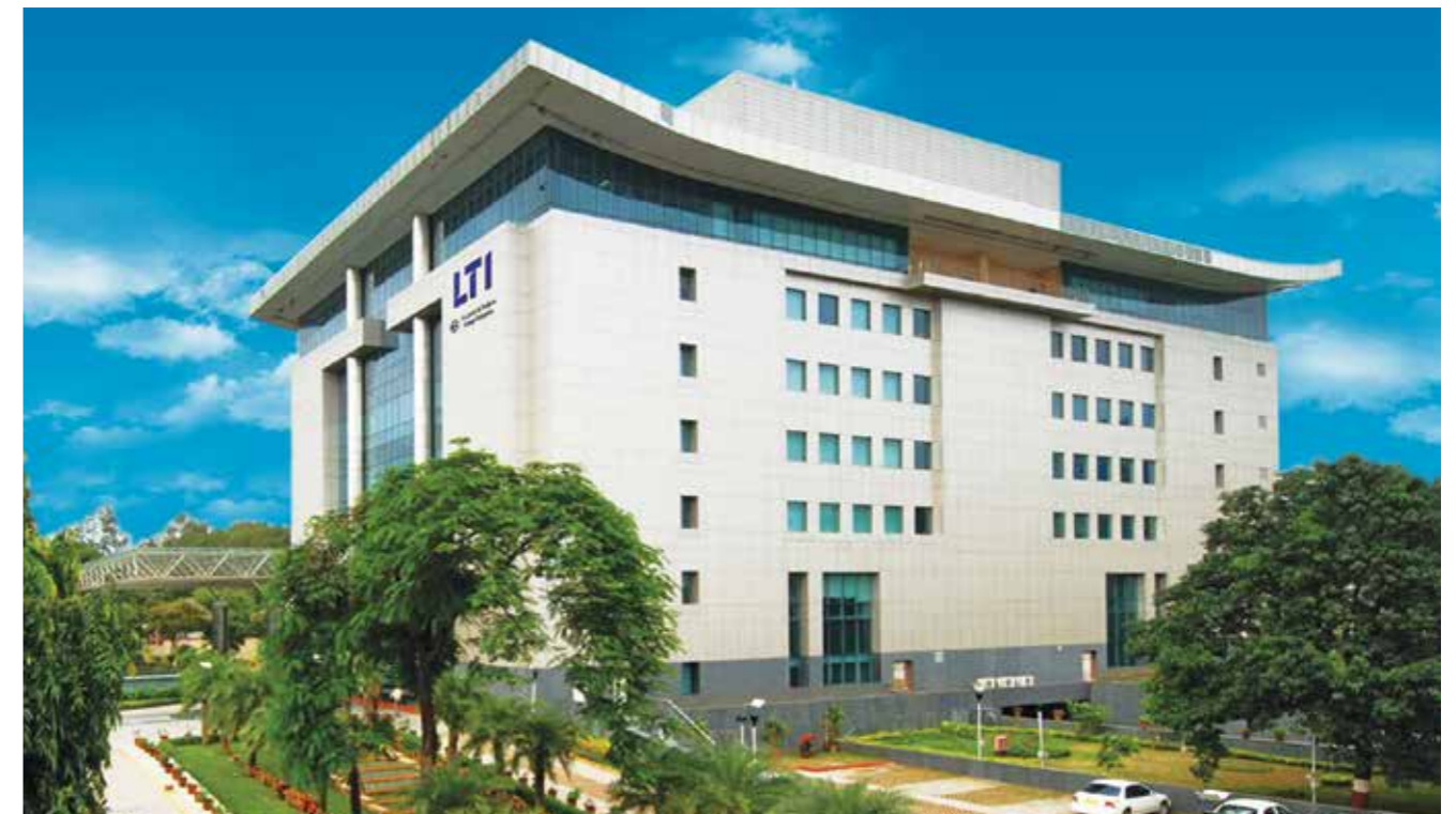
LTI's global headquarters in Powai, Mumbai
