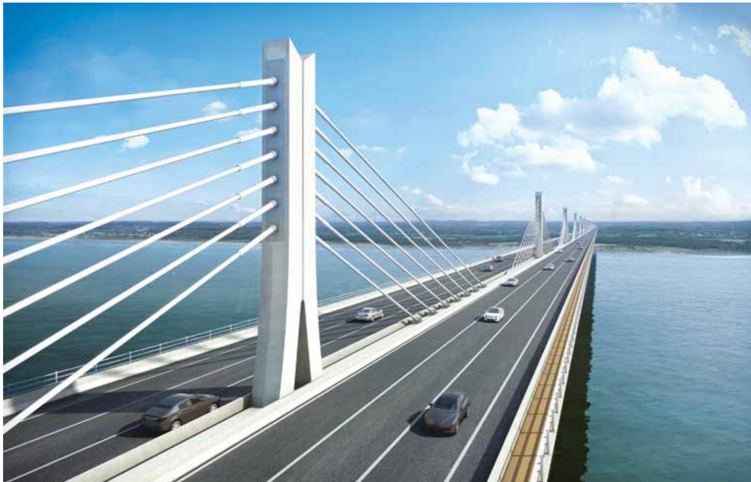
9.76 km Kachhi Dargah Bridge across river Ganga in Bihar, once completed, will be one of the longest extradosed river bridges in India
