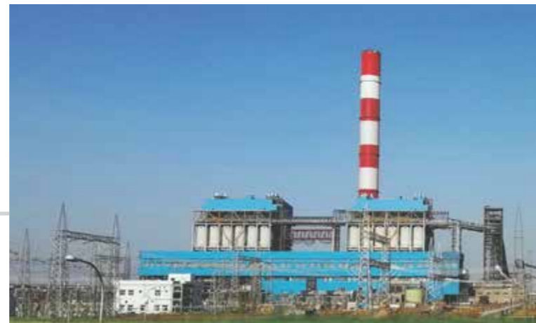
2x660 MW Shree Singaji Thermal Power Plant, (Stage-II) Madhya Pradesh
