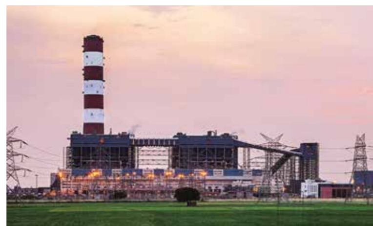
2x700 MW Rajpura Thermal Power Plant, Punjab
