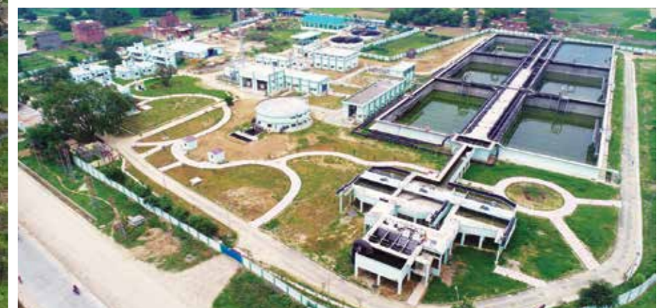
120 MLD Sewage Treatment Plant, Varanasi, Uttar Pradesh
