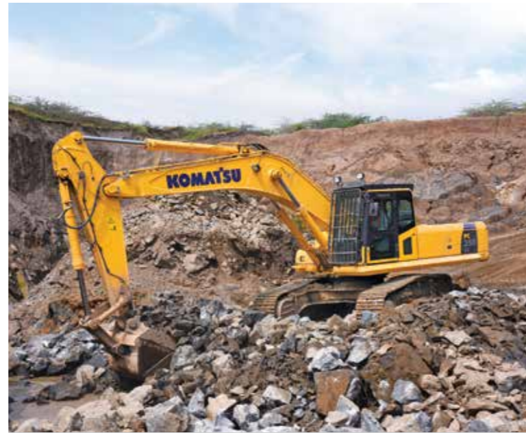
Komatsu PC350LC-8M0 Hydraulic Excavator
