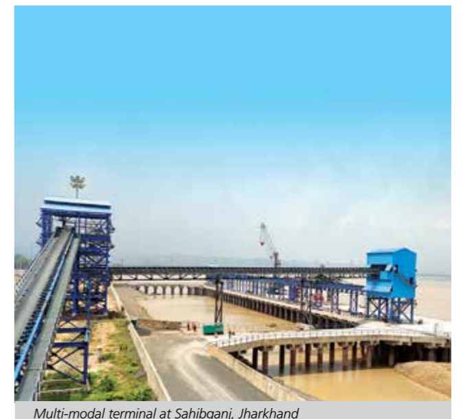
Multi-modal terminal at Sahibganj, Jharkhand
