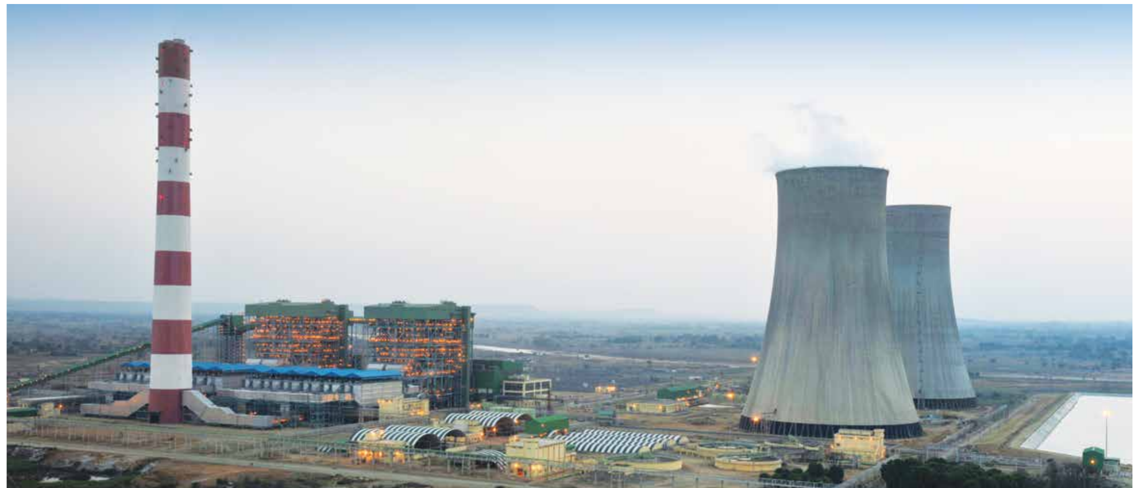
2x660 MW Jaypee Nigrie Thermal Power Plant, Madhya Pradesh
