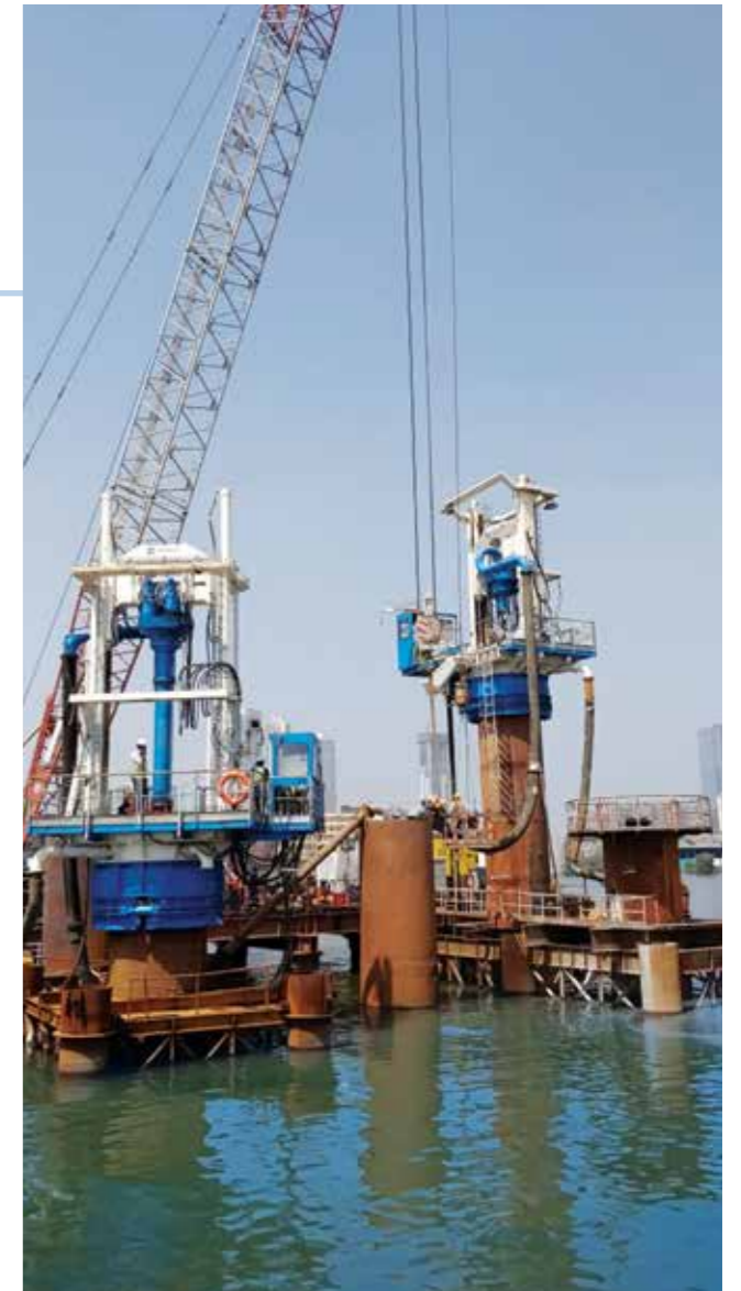
Reverse Circulation Drilling (RCD) rigs in operation at MTHL, Mumbai
