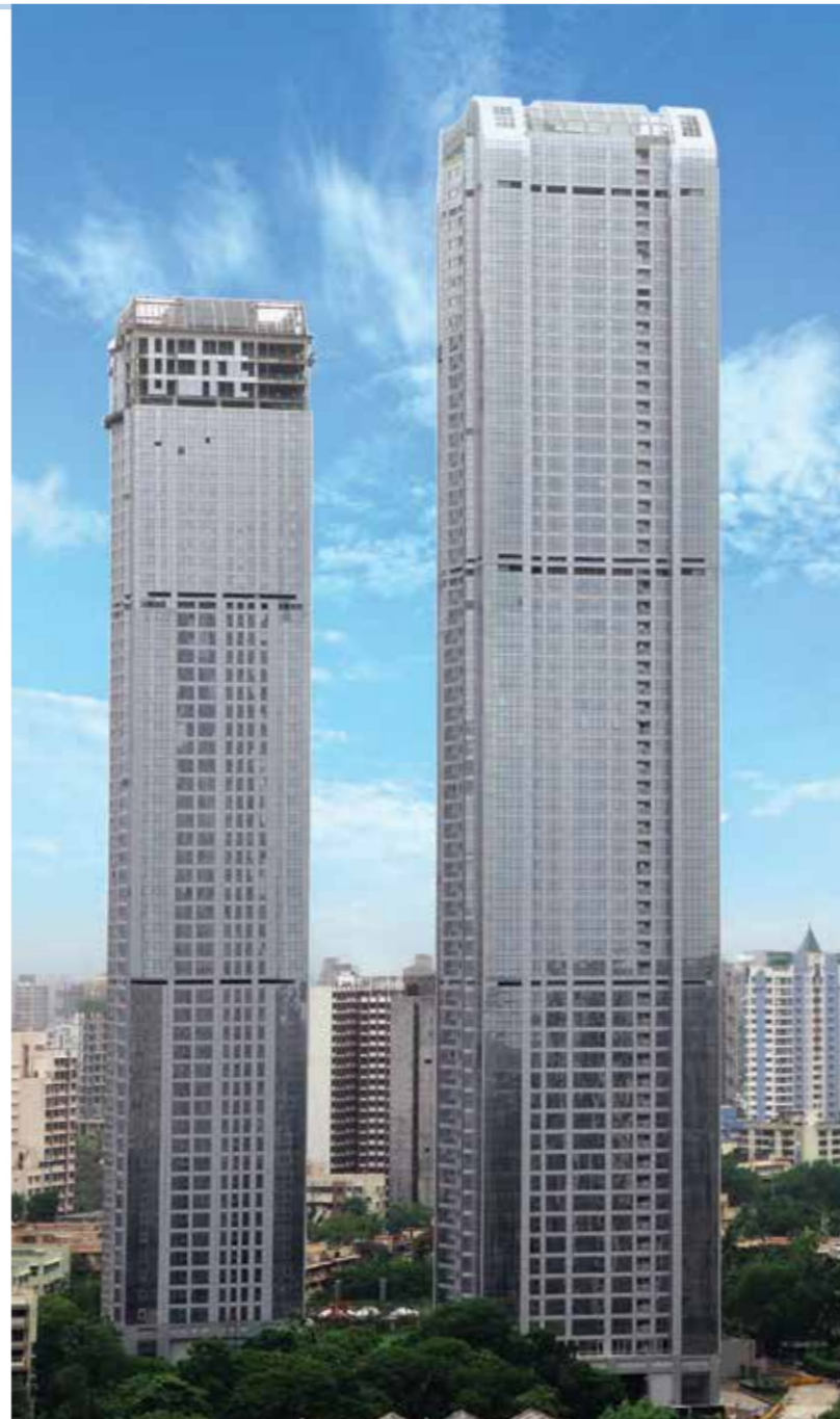
ICC Towers, Mumbai
