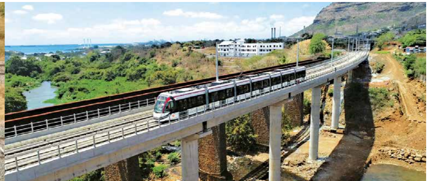
A section of the 13 km Phase 1 of the Mauritius Metro
