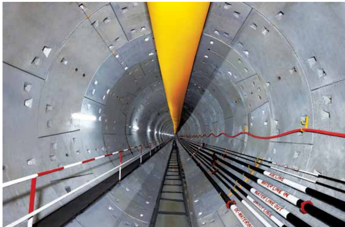
One of the underground tunnels of the Mumbai Metro project
