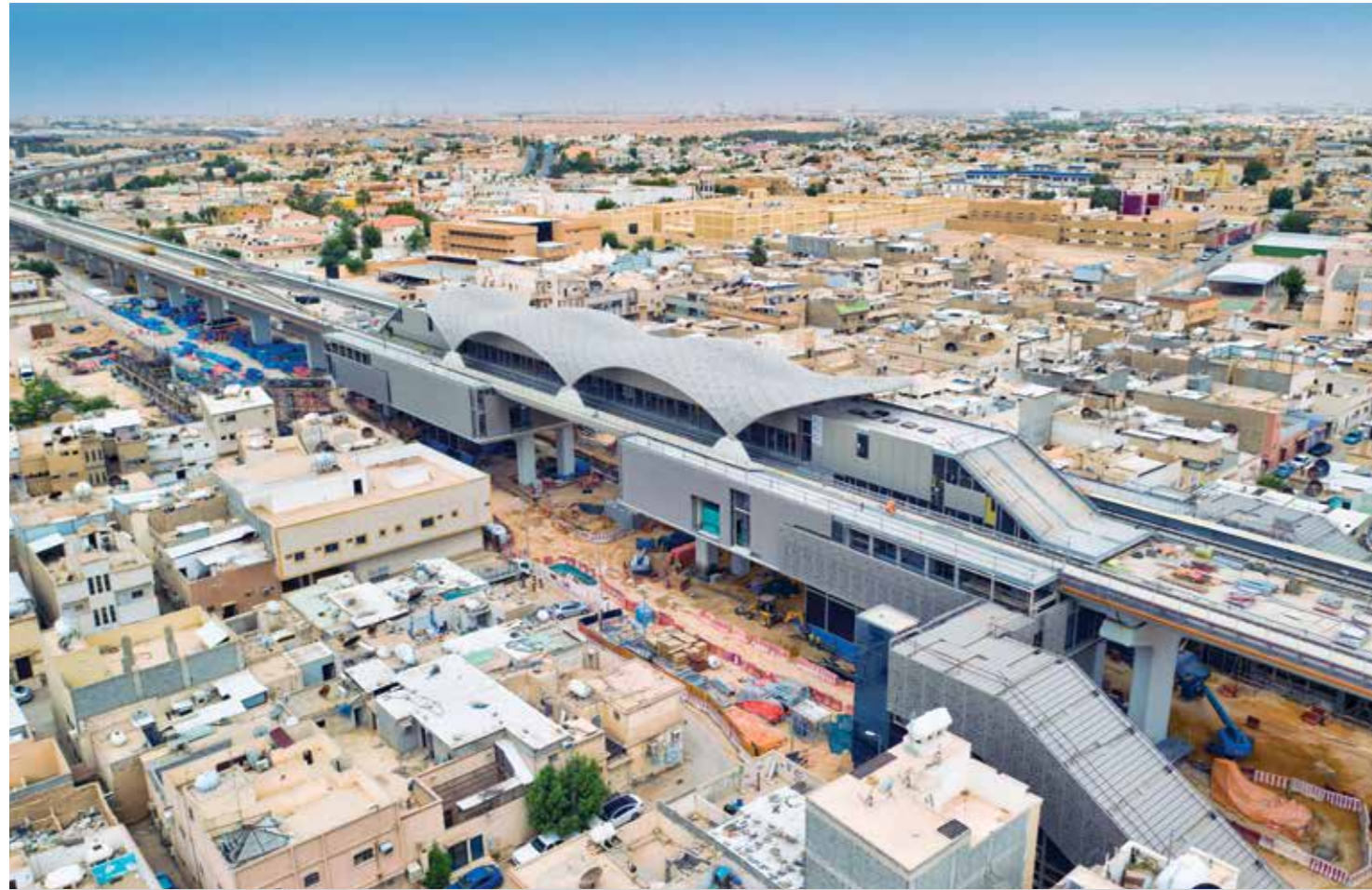
One of the stations of Riyadh Metro
