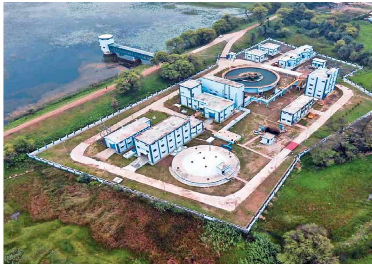
10.6 MLD Water Treatment Plant, Bagidora, Rajasthan
