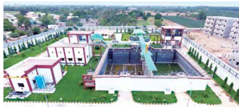
55 MLD Sewage Treatment Plant, Nellore, Andhra Pradesh
