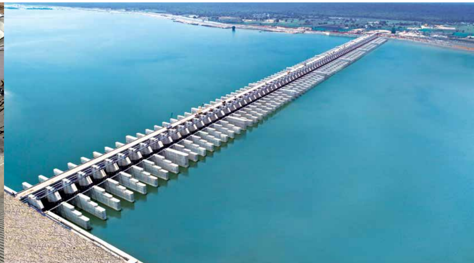
1.6 km Medigadda Barrage, Telangana, was built in a record 24 months
