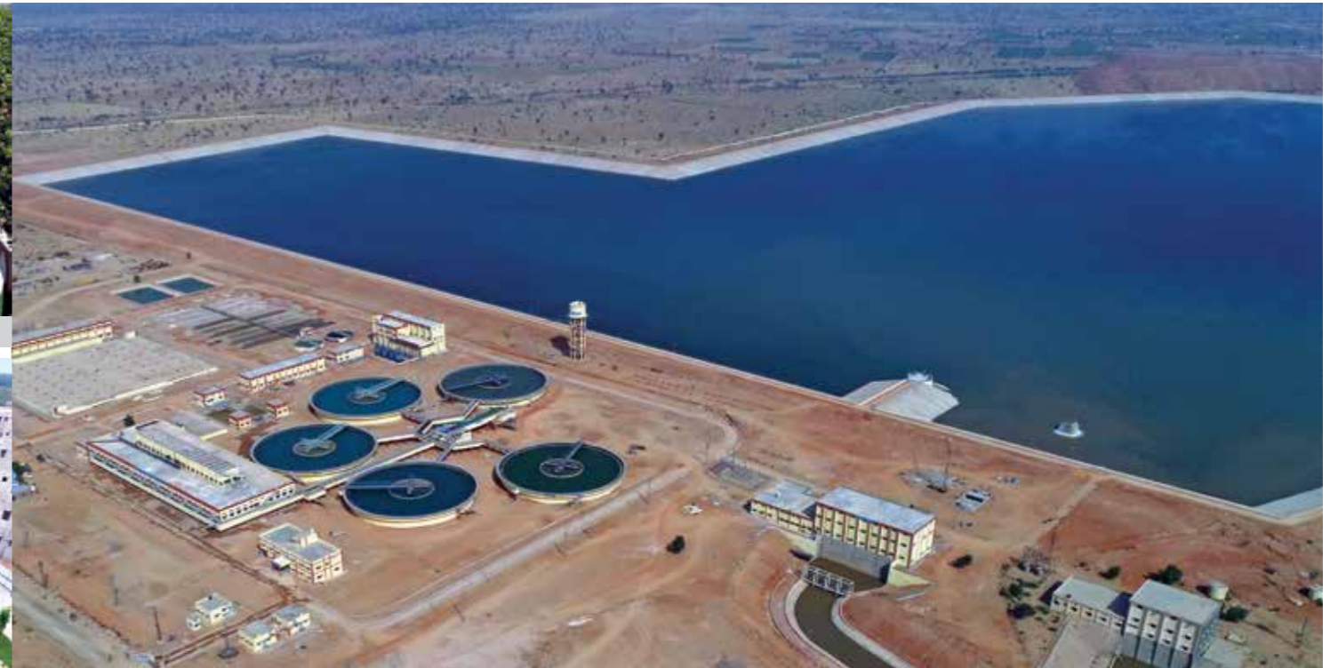
250 MLD Water Treatment Plant, Nagaur, Rajasthan
